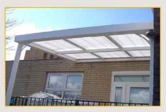
Each modular unit is designed to suit specific project requirements. Therefore on-site modification is significantly reduced. This system can be used as a replacement for old patent glazing and rooflight applications as well as offering an alternative to new canopies and walkways. Its modern design de-skills the installation process and is also capable of being manufactured to an infinite length with glazing centres generally 1015mm.
